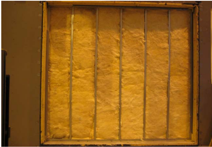
R-13 Insulation Installed in Cavity
